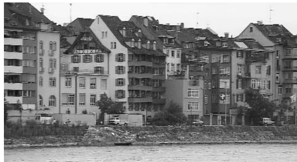
Fig. 6 Buildings along the Canal.
